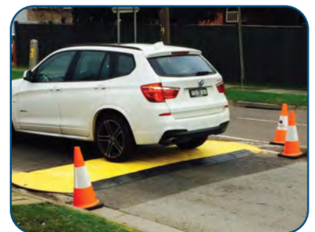
Ramp profile slows vehicles in work zones
