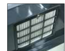
Internal air conditioner filter
